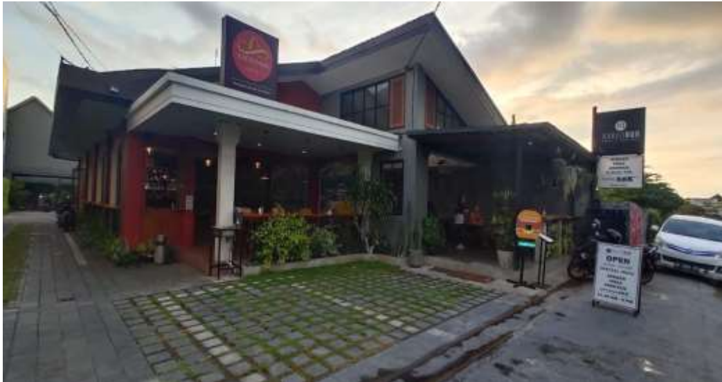
Figure 1. Taco Casa Canggu building (Source: Wijaya, 2021)
