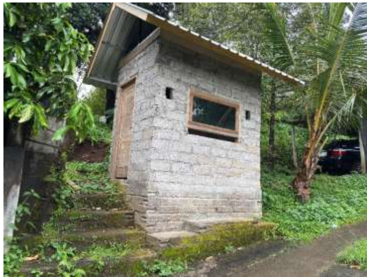
Figure 1. Condition of Wana Ayu Waterfall Guard Post (Source: Juniarta, 2025)
