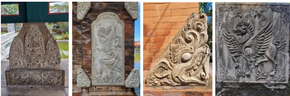
Figure 7, 8, 9, & 10. Balinese ornament with concrete molding technique [Source: Author's Personal Document, 2022]
