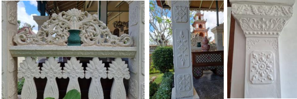
Figure 4. European ornament with concrete print technique [Source: Author's Personal Document, 2022]
