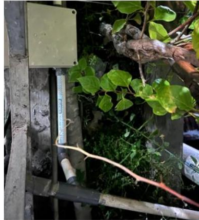
Figure 3. Physical Installation of the Campus Water Supply Line
